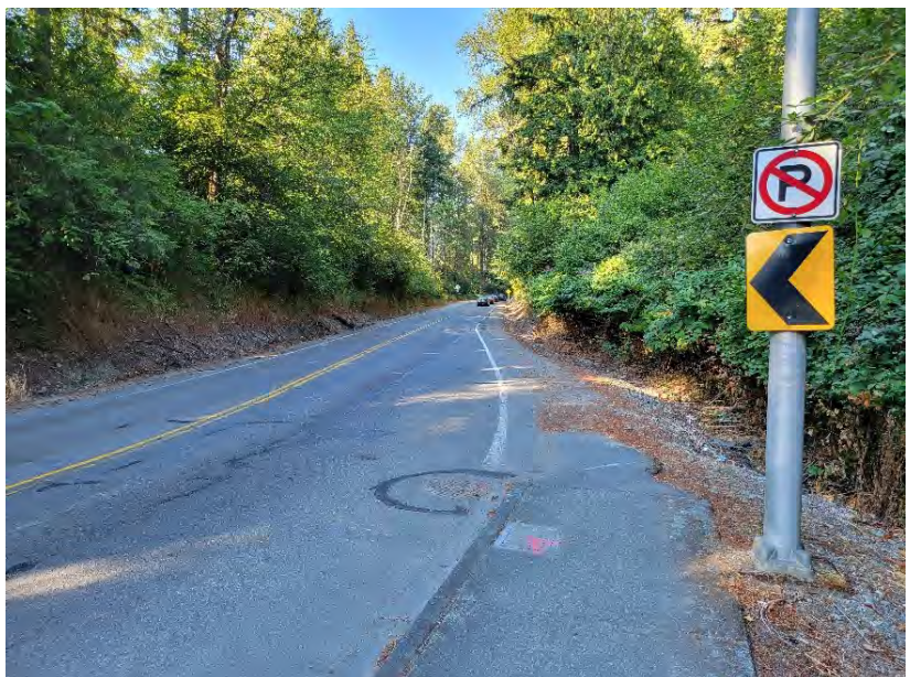
Typical view showing the portion of Riverwalk Drive without sidewalks
